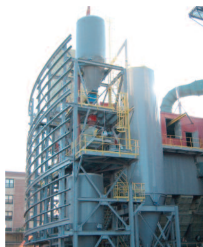
The second dry scrubbing system installed at Virginia Tech in 2007 is helping the school meet all state and federal emission requirements.
