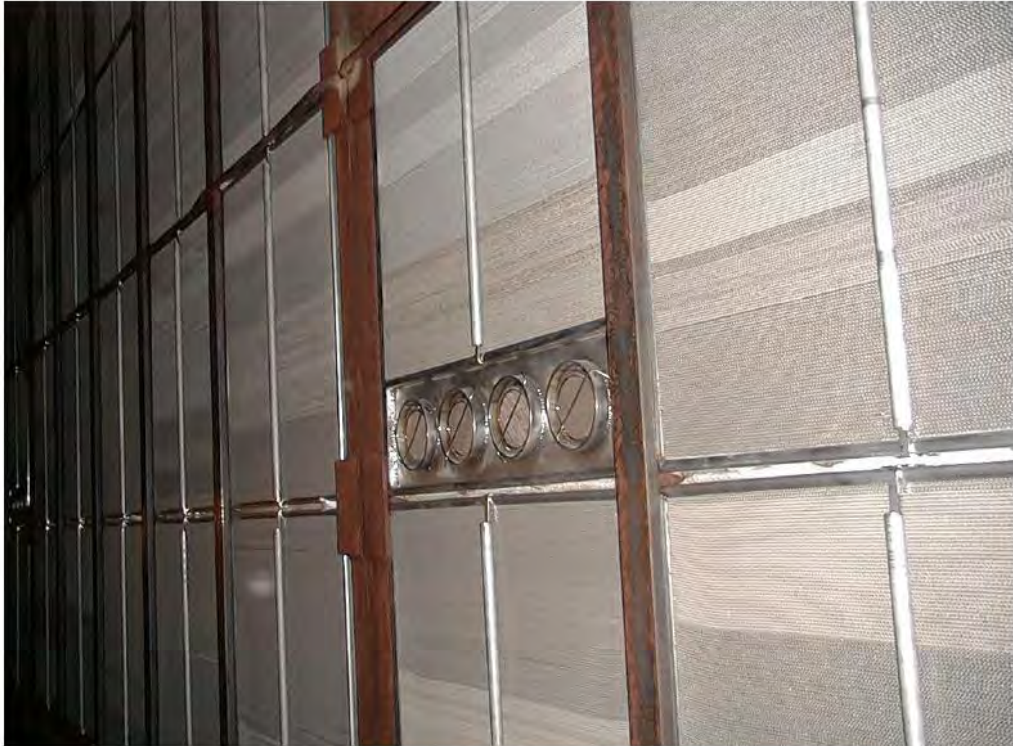
Figure 5. Monolithic Oxidation Metal Foil Catalyst Assembly (Source: Siemens HRSG O&M Plant Installation)
