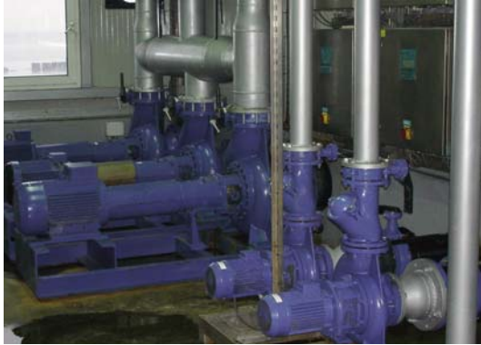
▲ Three ITT Vogel LS pumps with cast iron Duplex impellers and shafts. Two ITT Vogel LM series pumps back up and supply the smaller units.
