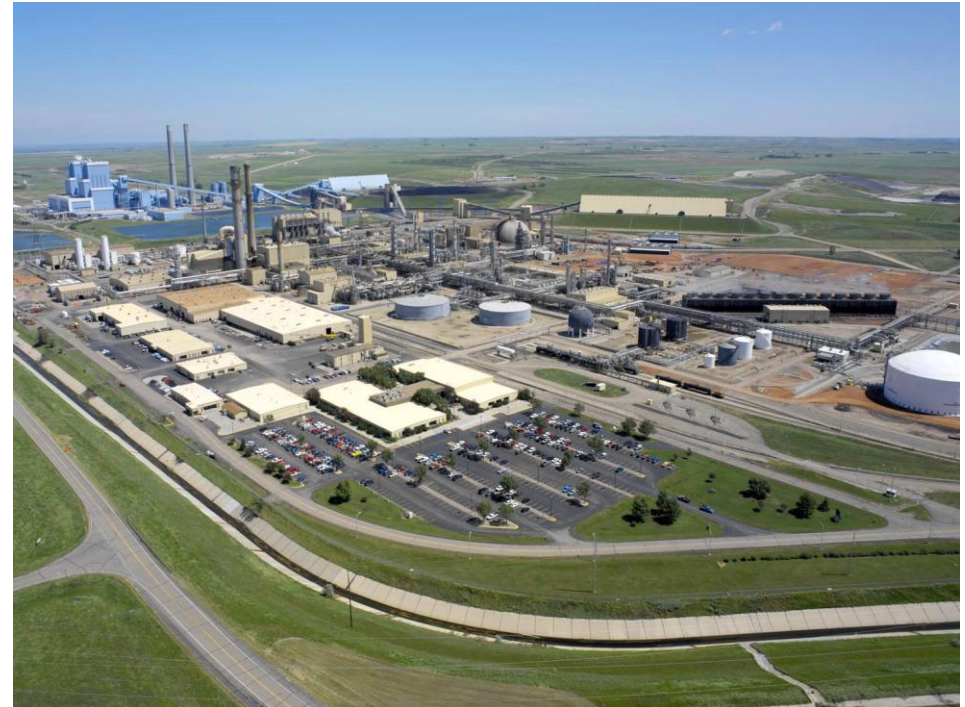
Basin Electric Antelope Valley Station (in background) and Dakota Gasification Facility (in foreground)
