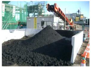
Photograph 11. Discharging dewatered sediment
