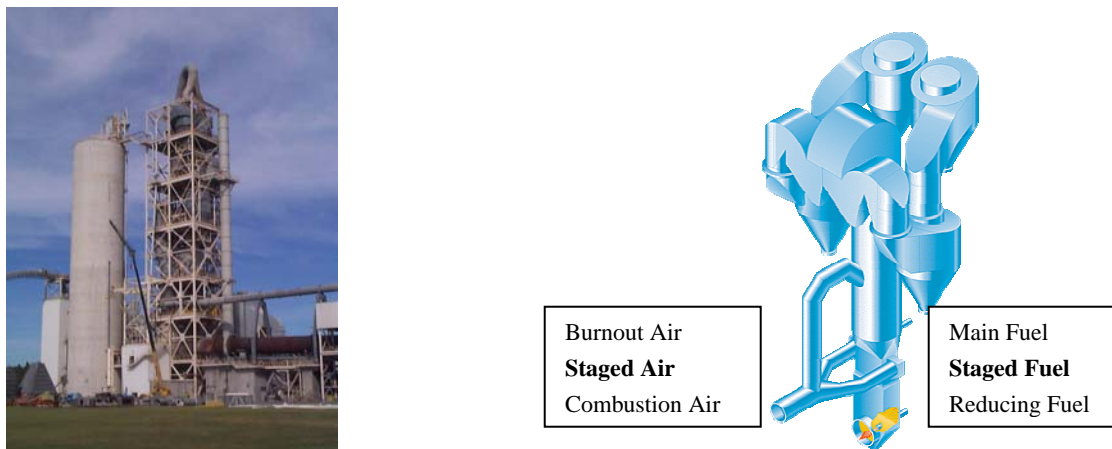
Figure 2. Florida Rock Industries PH/C Kiln and Diagram of Fuel and Air Staged Calciner
