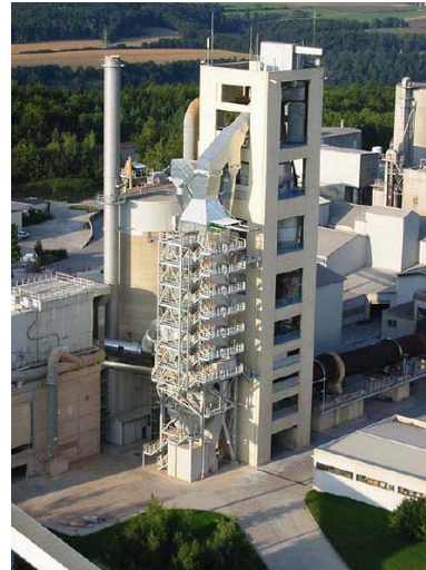
Figure 14. SCR System Adjacent to Preheater Tower at Solnhofer Portland Cement Plant.
