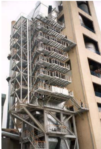
Figure 14. SCR System Adjacent to Preheater Tower at Solnhofer Portland Cement Plant.
