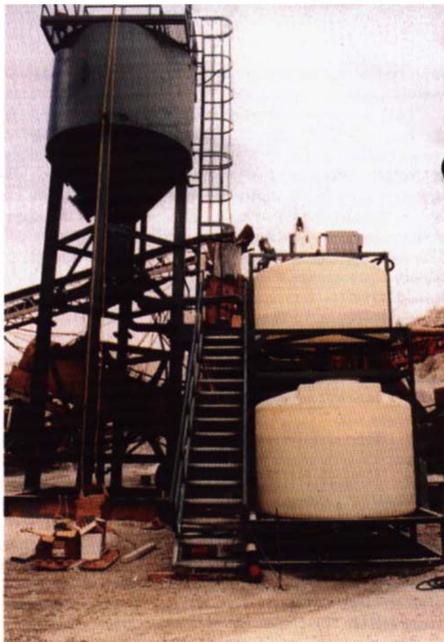
This Aqua Clear clarifier processes dolomitic limestone fines of which 80% pass the 600 mesh at a plant in Illinois.
