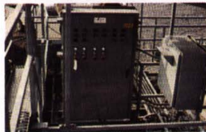
Output from the Jadair clarifier (above) is controlled by a solid-state electronics/microprocessor package (right).
