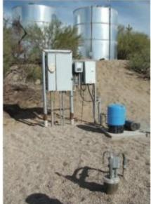
The water source comes in the form of two 10,000-gallon storage tanks – each fed by a submersible pump in a deep water well installed and serviced by Walt Kadle, a Goulds professional dealer.
