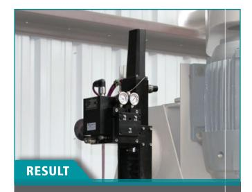
Upgrading from pneumatic actuators to REXA Electraulic<sup>™</sup> Actuators on boiler feedwater recirculation valves can provide immediate benefits for any power plant. Maintenance savings can be immediately realized through tighter shut-off, improving trim life of the control valve, and reducing labor and material costs.
