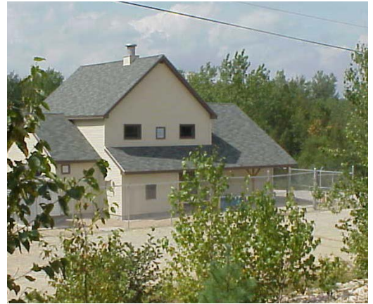
Town of Raymond water treatment plant.
