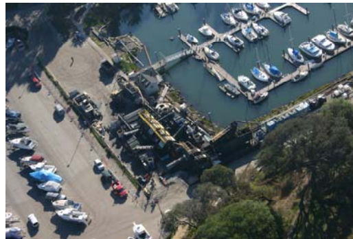
Figure 2. Rapid dewatering facility at Santa Cruz Harbor
