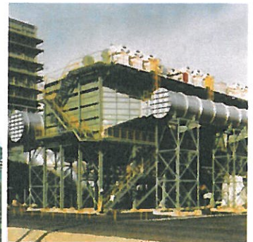
• Wet Type Horizontal Flow ESP
