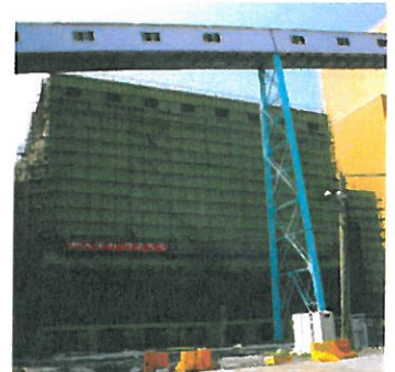
• Taichung Steam Power Units 9, 10 ESP
