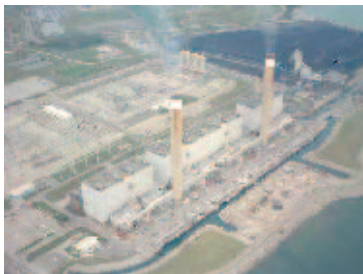
The Nanticoke plant is a coal-fired power generating plant, located on the north shores of Lake Erie, Canada.
