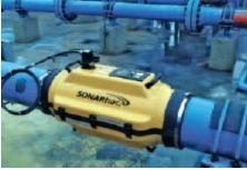
CiDRA's SONARtrac flow technology is an industrial flow meter, using measurement principles that are distinct from all other flow meter technologies operating in mining. SONARtrac non-intrusive flow monitoring systems make no contact with the slurry and can be removed and reinstalled without process interruption.
