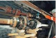
Paterson & Cooke has developed some specific technologies, like the patented Energy Dissipator (ED). Its function is to control the flow rate and hydraulic profile in piping systems with significant changes in elevation.
