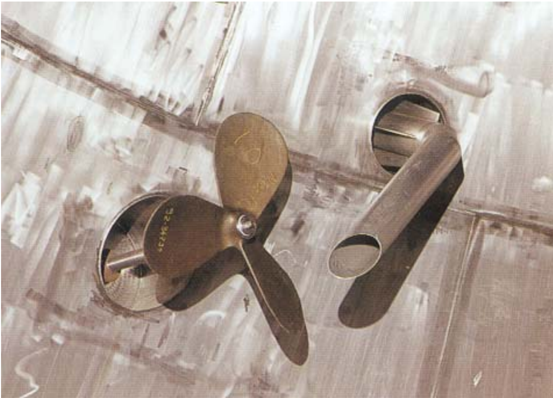
Figure 20: Oxidation Air Lance and Agitator Impeller
