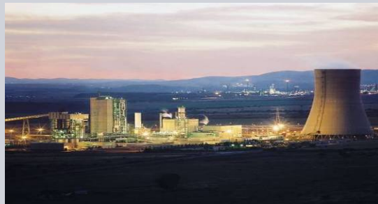
Siemens IGCC technology applied in Puertollano (E)
