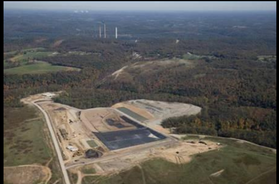
Dry Storage = nonhazardous
