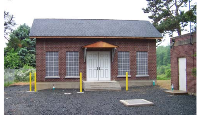
This is the building that was erected around the Liqui-Cel® Degassing System. This installation is in a residential area and it was important to conceal equipment in an aesthetically pleasing manner.
