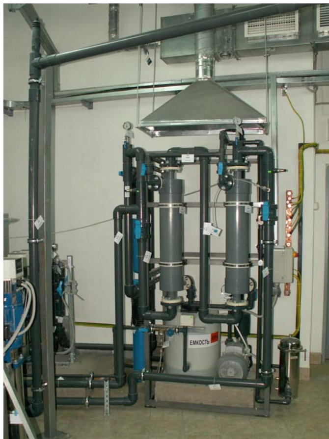
Liqui-Cel® Water Degassing System used at the Ice Palace to produce Crystal clear ice at the arena
