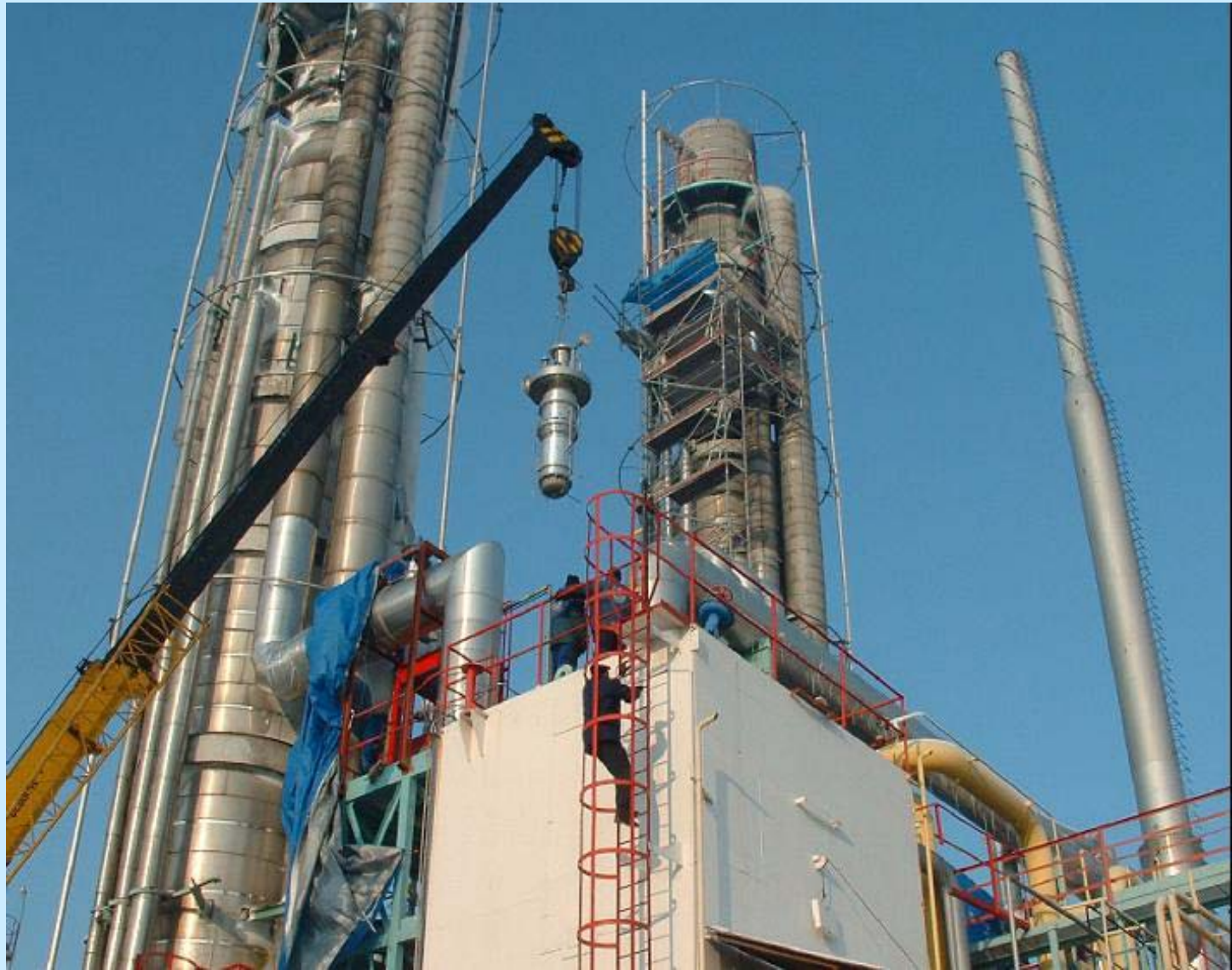
Installation of the Very First Two-Phase LNG Expander in Poland 2001
