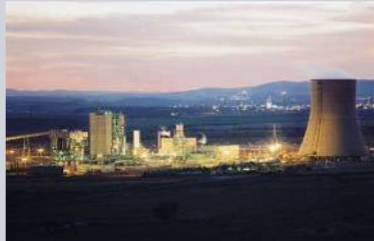
Siemens IGCC in Puertollano (E)
