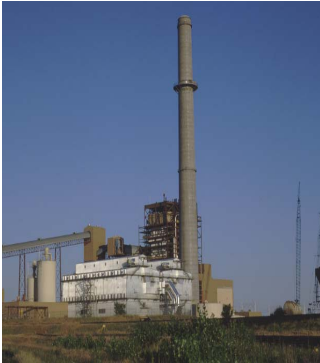
Public Service Company, Colorado Pawnee Station, Unit 1, 550 MW
