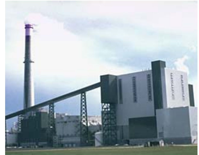
Orlando Utilities Commission Stanton Units 1&2 - 2 x 465 MW Orlando, Florida
