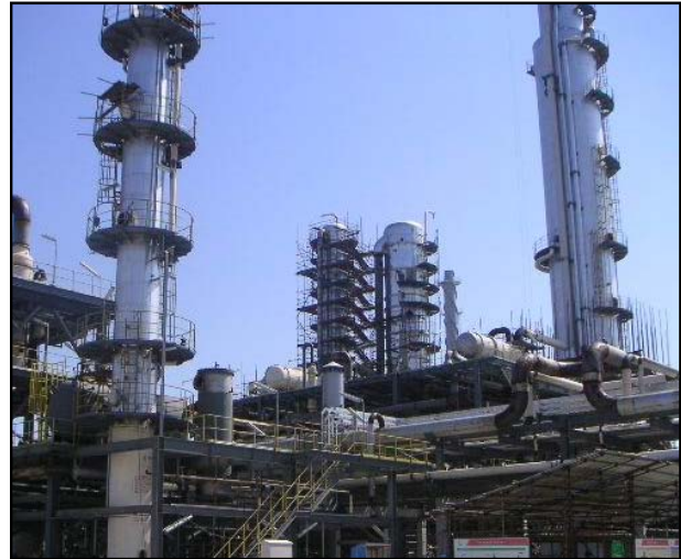
Shanghai SECCO Acrylonitrile project plant
