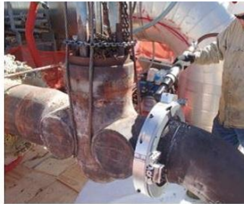
4. Valve is separated from 12-in. main steam piping
