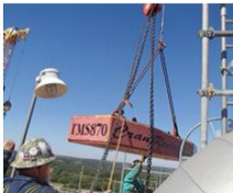
8. Safety first! Jib crane is load tested prior to use
