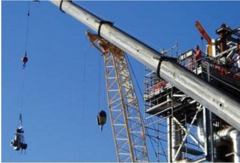
10. New valve is delivered for installation
