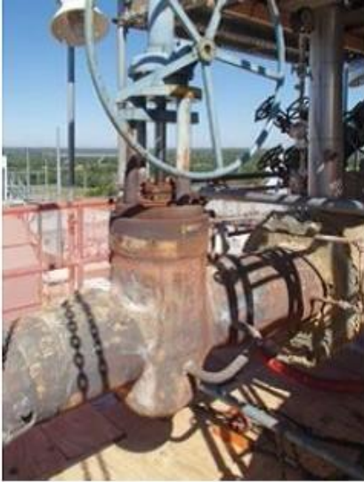
2. Original valve after insulation was removed
