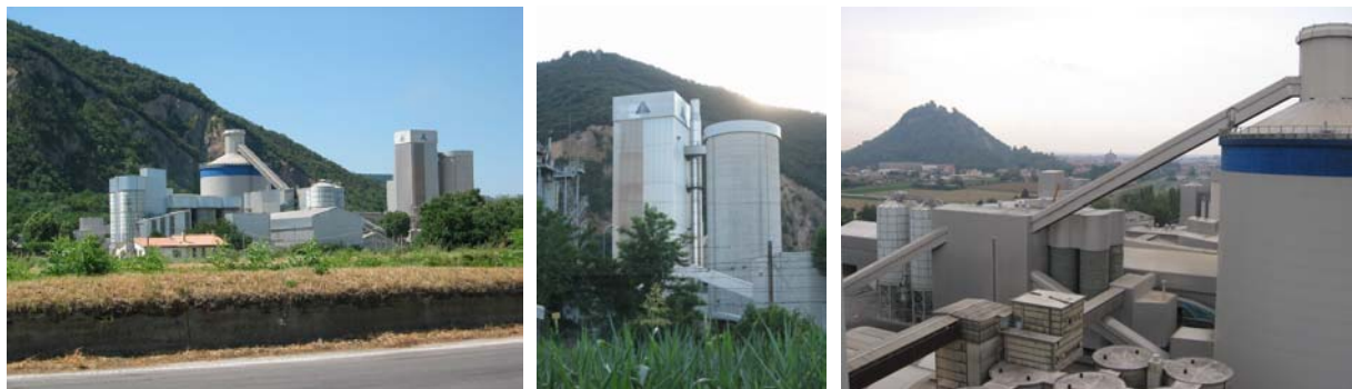
Figure 2. Photograph of CM from East. Preheater, Feed Silo, Stack. La Rocca from the Stack.
