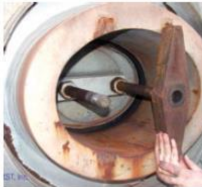
5. Proper gasket alignment is critical to a tight seal between HP drum access door
