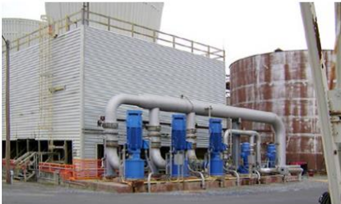
Main and auxiliary circ-water pumps overhauled
