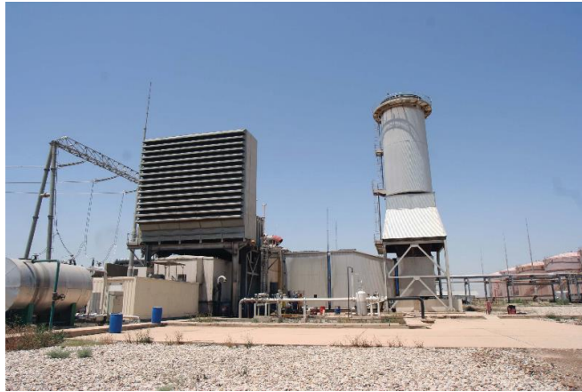
FIGURE 4. A example of a very large gas turbine installation. The air inlet filter and the exhaust gas stack are also shown.
