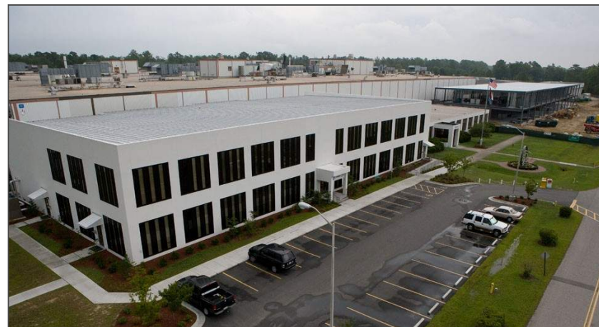
Advanced Technology Center
