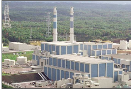
●Hokuriku Electric Power Co. Shika NPS
