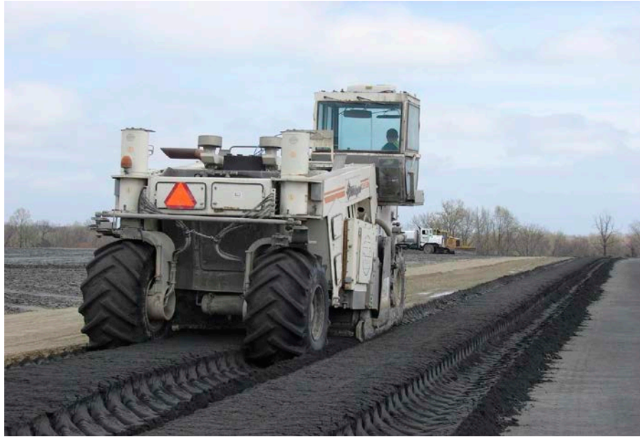
Figure 5 - Reagent Mixing Operations on CCP with Trona™
