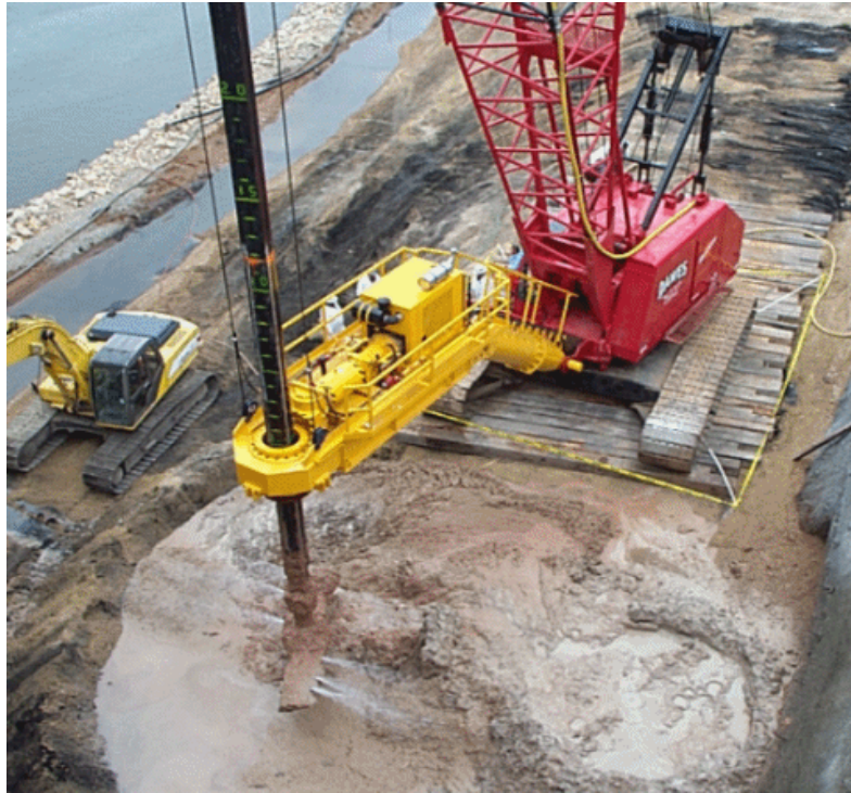
Figure 2 – Large Diameter Auger Mixing Using a Crane Mounted Drilling Platform
