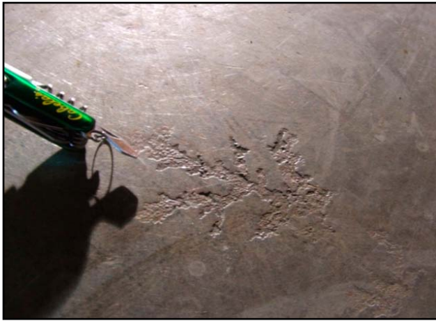
Fig. 2 Less severe surface etching.
