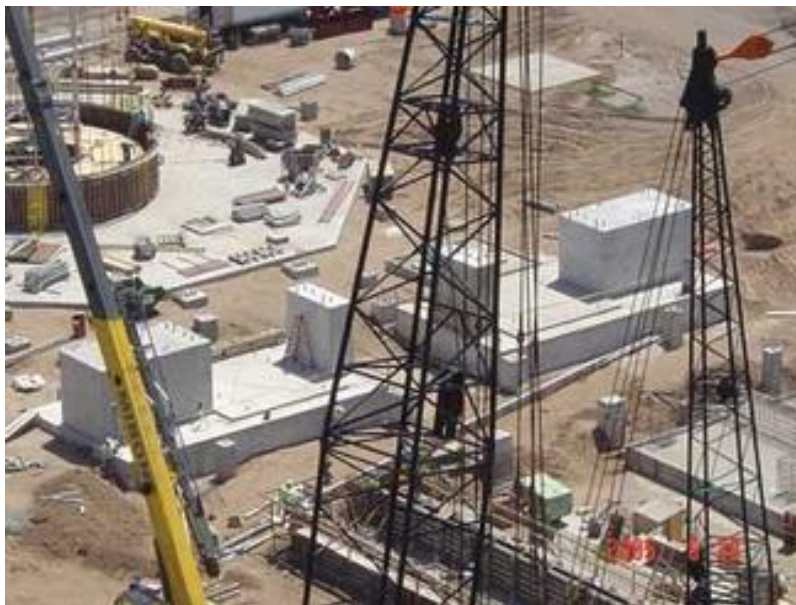
Induced draft fan foundations. Photo courtesy WPS.
