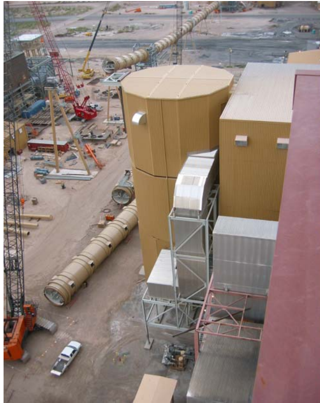
Figure 11. Springerville Unit 2 Spray Dryer Installation
