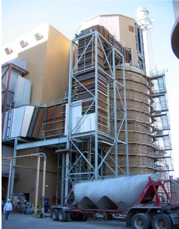
Figure 10. Springerville Unit 1 Spray Dryer
