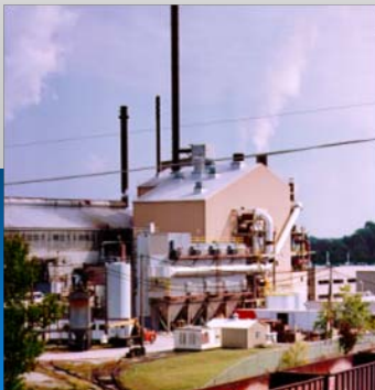
30 MWth Test Facility
