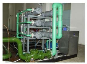
A Liqui-Cel® Contactor System built for Boiler Degassing by Shen Lan
