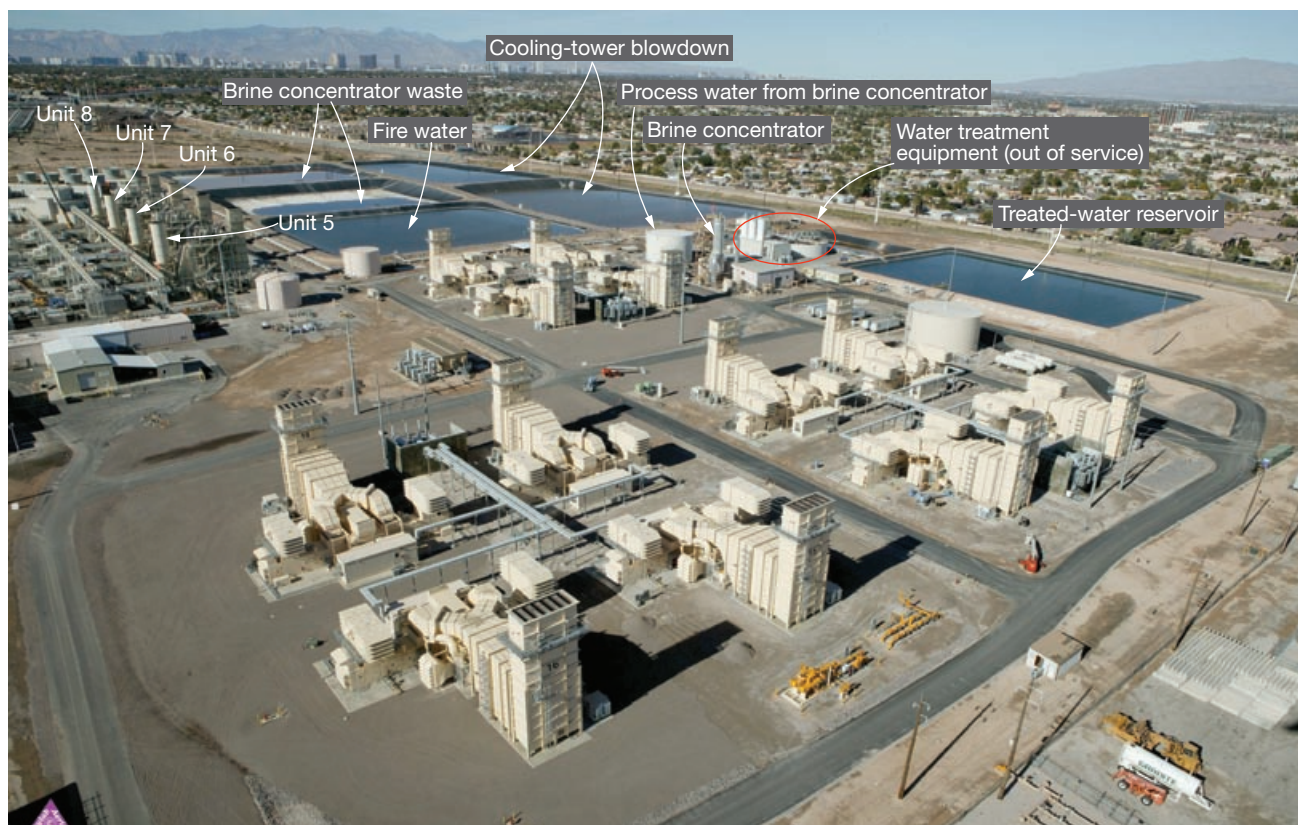
Clark Station is located with the city limits of Las Vegas. When the first steam/electric unit began commercial operation in 1955, the plant stood all alone in the desert. No city would have been visible in an aerial photo like this one. Today the plant is surrounded by an interstate highway, commercial buildings, and residential neighborhoods. You can even see the hotels and casinos on Las Vegas Blvd on the horizon. The company’s first three steam units were demolished to make room for the 12 SwiftPacs, arranged in three blocks of four units each at the bottom of the photo. Two combined cycles incorporating the four rehabilitated 501B6s (Units 5-8) are at the upper left
