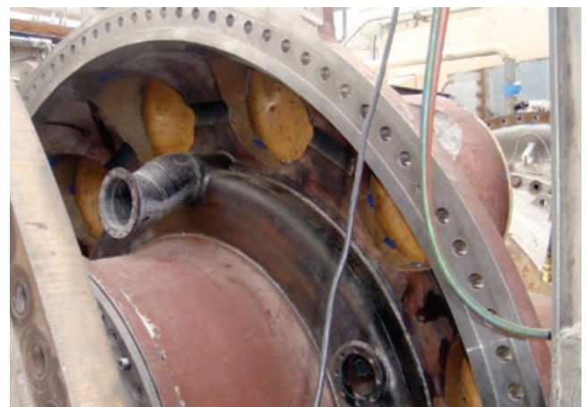
4-24. Upper-half casings replaced
