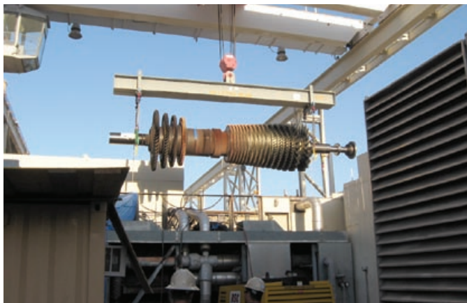
4-11. Rotor was removed and sent to shop for refurbishment
