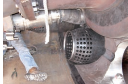
4-26, -27. Flow sleeve installed in CC case
