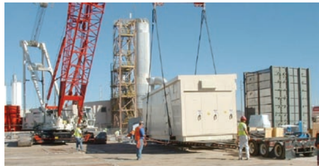
4-44. Control cab is lowered into position
