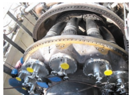
4-32. End covers installed
