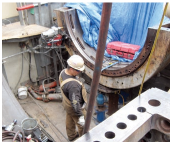
4-17. Millwright checks area after removal of OEM's CC case
