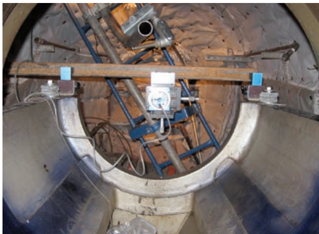
4-21. Alignment rechecked with new CC case installed
