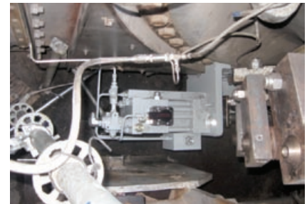
4-36. Hydraulic IGV actuator replaced the pneumatic one in Fig 4-35
