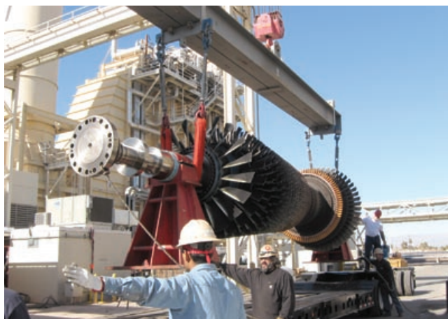
4-23. Upper-half casings removed once again and reconditioned rotor installed
