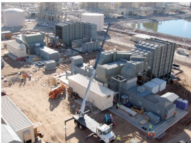
4-45. Erection progresses quickly. Major components and most ductwork are in place
