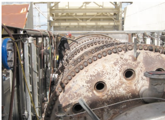
4-13. Upper-half casings reinstalled for casing alignment check
