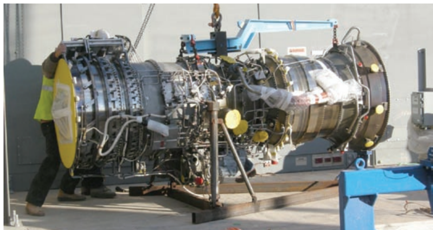
4-49. FT8-3 is unwrapped and prepared for installation
