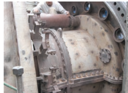
4-10. Rotor air cooling pipe visible after removal of combustion components
