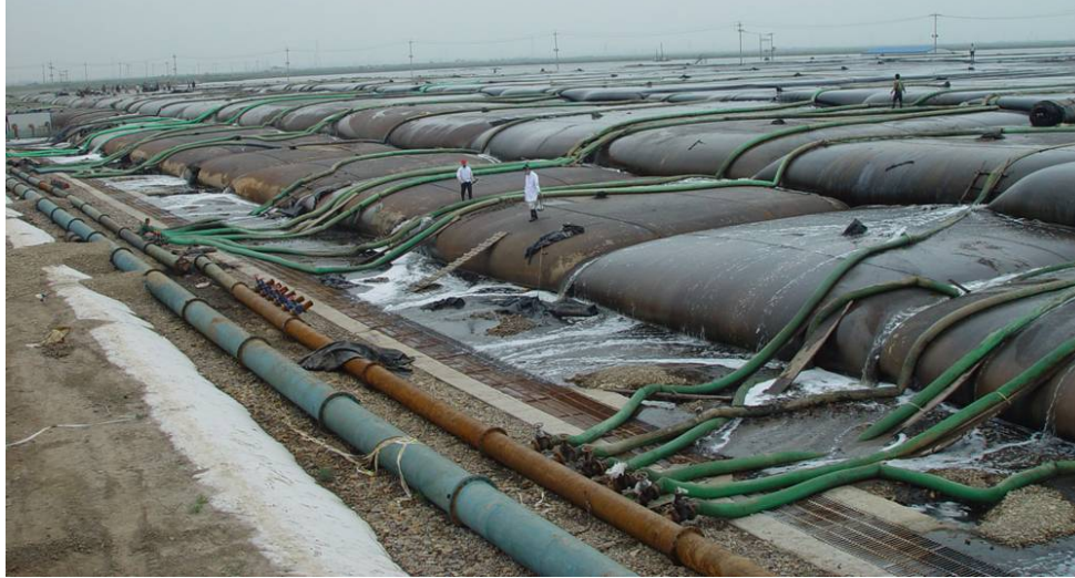
Figure 26. Overall view of geotextile dewatering work.
