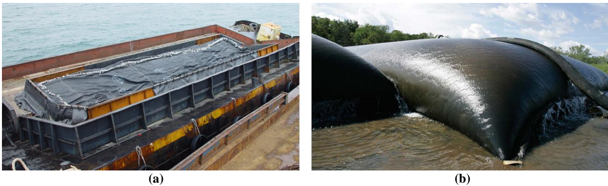
Figure 2. Geotextile containment solutions (a) geotextile container drop (b) geotextile tube dewatering application.
