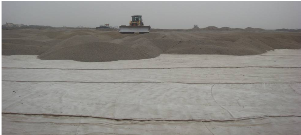
Figure 25. Backfilling of sand over reinforcement geotextile.
