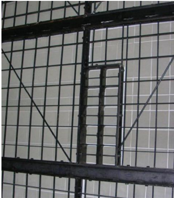
6. Take a quick sample. A sample tray installed on a catalyst module enables taking a catalyst sample very quickly. Courtesy: Cormetech Inc.
