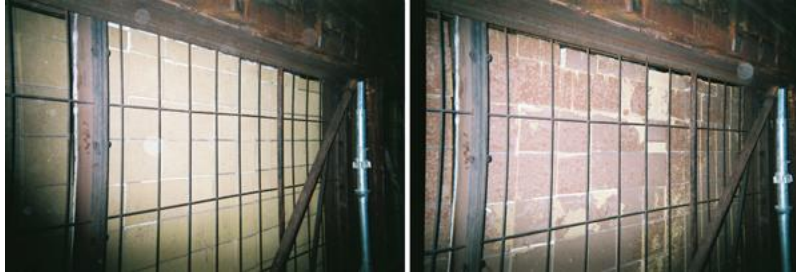
4. Keep your catalyst clean. Ash and other contaminants can blind the insulation layer around the catalyst. Shown are the catalyst modules when clean (right) and when the catalyst performance is reduced by blinded insulation (left). Courtesy: Cormetech Inc.
