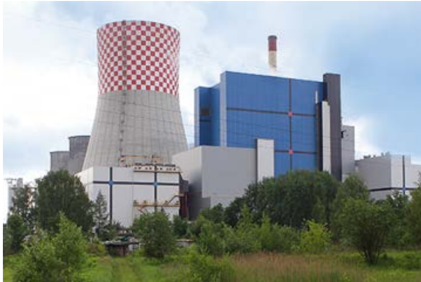
Figure 1. Lagisza CFB Power Plant located in Bedzin, Poland
