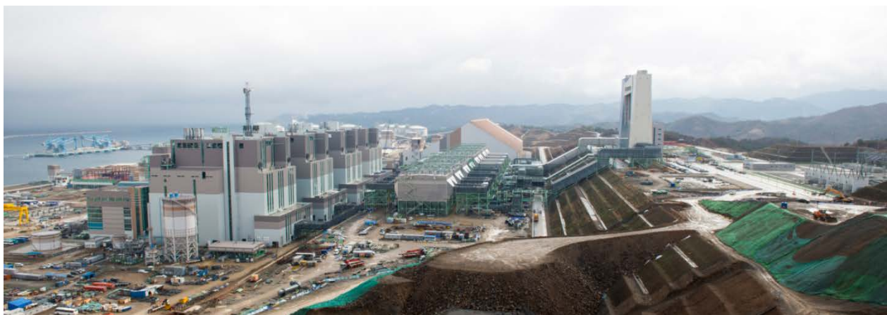
Figure 2. The 2,200 MWe Advanced Green Power CFB Plant in Samcheok, South Korea
