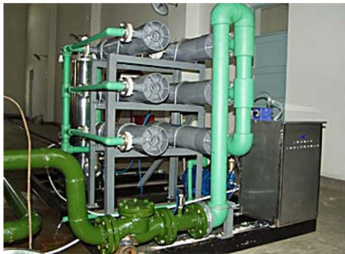
*Membrane Contactor Boiler Deoxygenation System built by Shen Lan*
