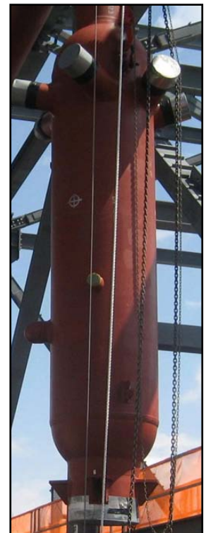
Fig. 16 Vertical separator.
