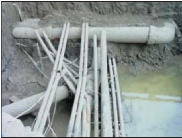
Fig. 11 Underground exposed obstructions during Hydro-Vac excavation.
