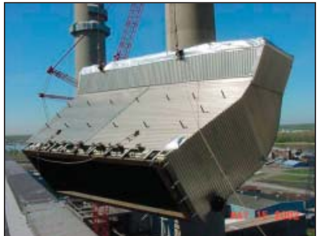
Fig. 15 Pre-assembled SCR flue shown during installation, complete with insulation and lagging.
