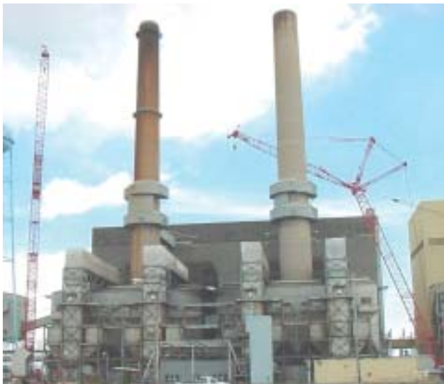
Fig. 1 D.E. Karn Units 1 and 2 during SCR installation
