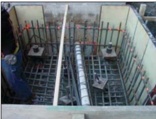
Fig. 12 Typical micro-pile installation.
