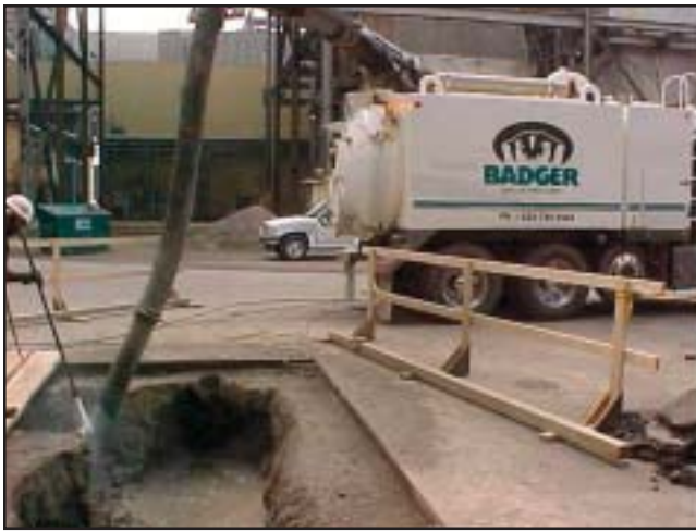
Fig. 10 The Badger Hydro-Vac “soft-dig” excavation technique safely exposes underground obstructions.
