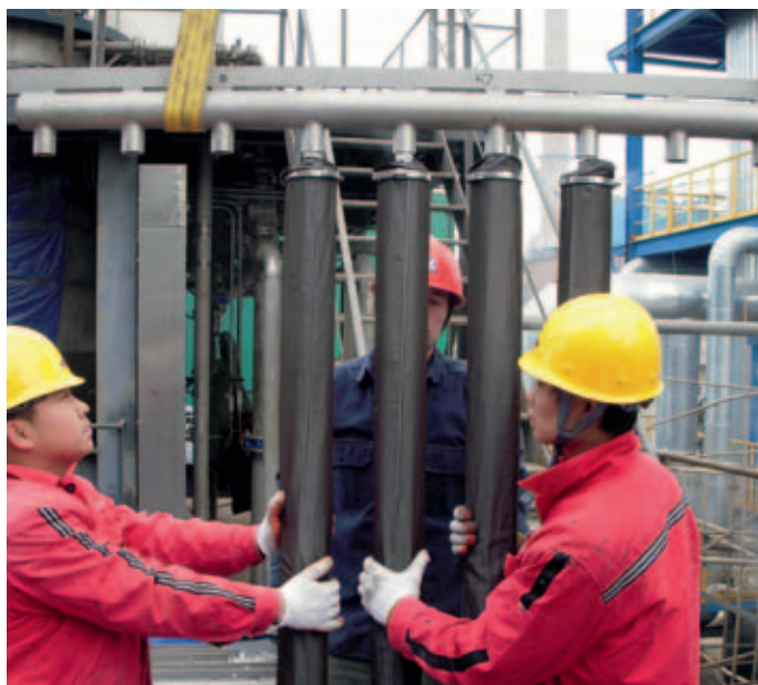
Installation of a BHS candle filter system at site.
