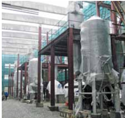
▲ Shanghai sewage treatment plant, Bailonggang, during the building phase
