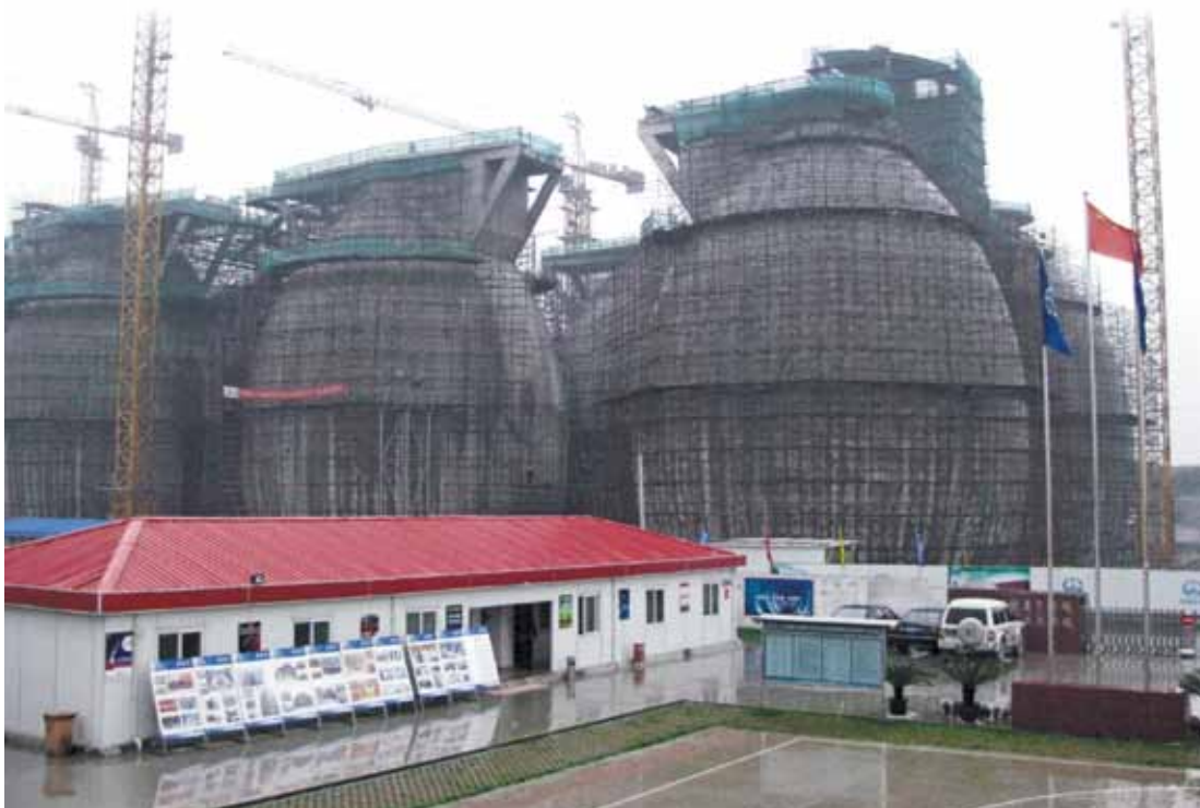
◀ Shanghai sewage treatment plant, Bailonggang, during the building phase
