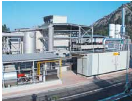
▲ BDS plant in Antalya, Turkey, gas motor + dryer
