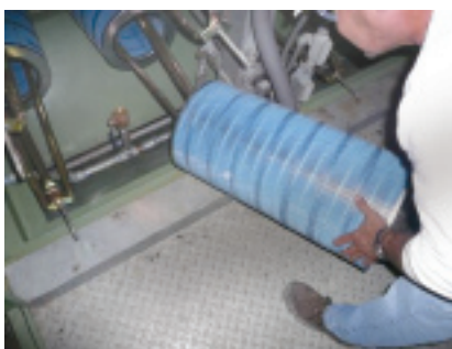
6. A pulse-type filter , typically specified for dry environments, is installed
