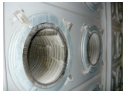
14. Pleated prefilter protects HEPA from large particles
