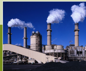
TRC performed mercury testing at the coal-fired Four Corners Power Station in NM.
