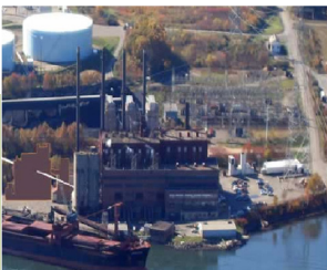
TRC utilized the Ontario Hydro Method for mercury testing at the Schiller and the Merrimack Stations in NH.
