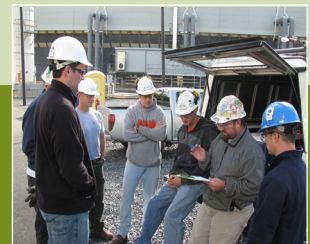
Safety is first at TRC; toolbox talks are performed at the beginning of each shift.
