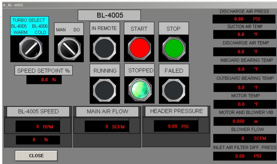
Figure 10 - Control Room Operation Screen
