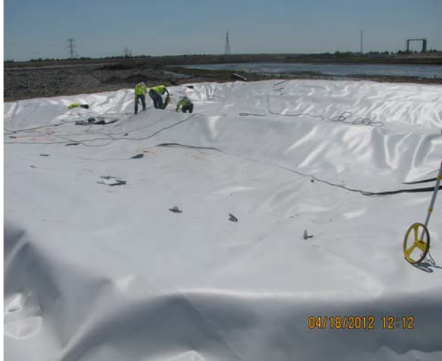
Figure 7- Geomembrane Installation
