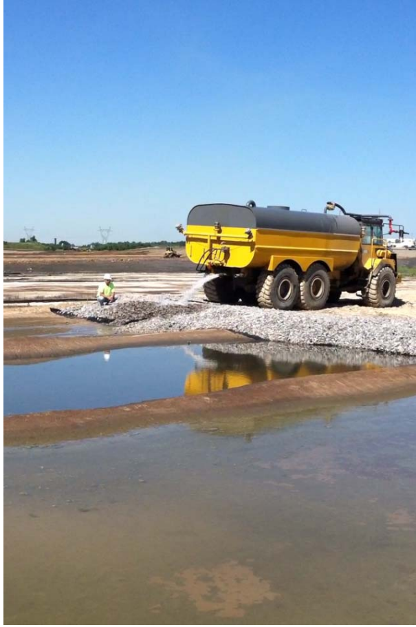
Figure 11 – Water Truck Dosing
