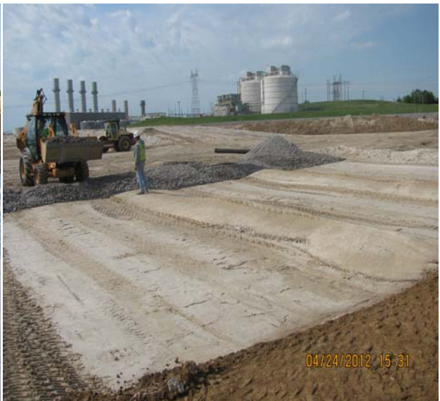
Figure 10 – Gypsum Placement
