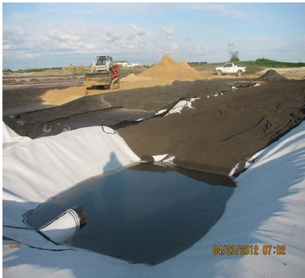
Figure 9 – Ash Placement
