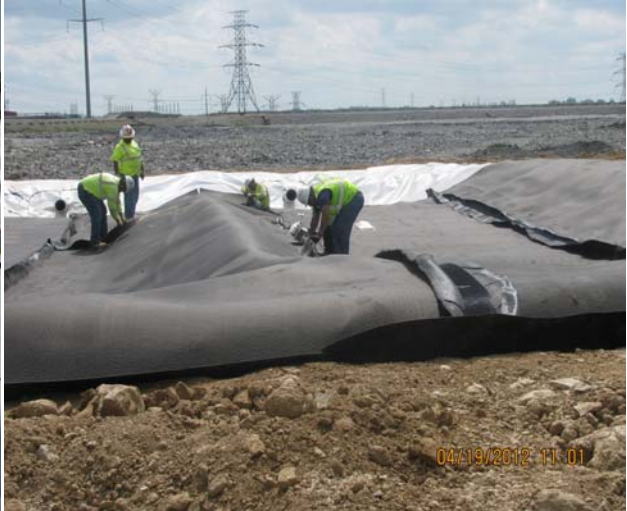
Figure 8 – Geocomposite Installation
