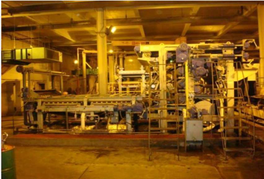
North WWTP (2-m)
