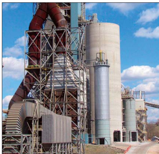
Lehigh Cement plant in Union Bridge, Maryland. (Photo courtesy of Lehigh Cement. 2006.)
